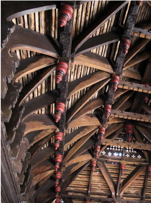
Figure 11. Roof structure. Image: Gopika Jayasree
