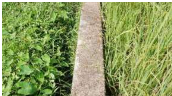
Figure 6. The varambu , or levee, that divides the smaller plots in a paddy field is made of concrete instead of mud in Justin’s field. Image: JANAL Archives, 2024
