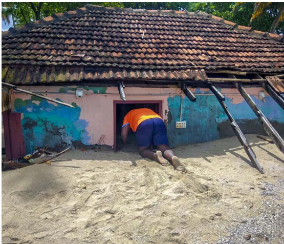
Figure 5. Man clearing the slit from a house ravaged by the flood. Photo taken during the restoration process after the flood. Image : George Babu, 2022.
