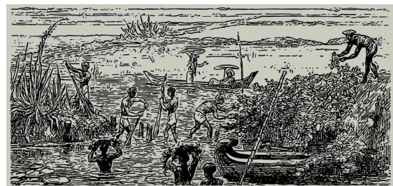
Figure 2. Repairing the bunds or kayal. Image: illustration from the magazine The Graphic , April 1877.
