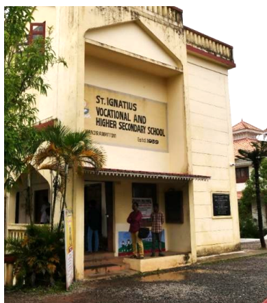
Figure 1. St. Ignatius VHSS, Kanjiramattom. The vocational school began in 1991, while the vernacular school started in 1939. Image: JANAL archives, 2023
