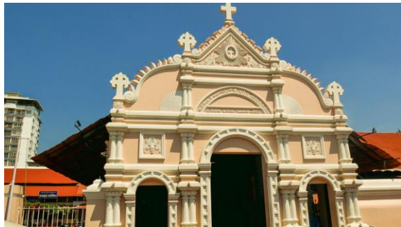
Figure 3. The Marth Mariam Valiya Palli was built in 1814 by the Chaldean traders of Thrissur, who came to the city in 1796. Image: JANAL Archives, 2024
