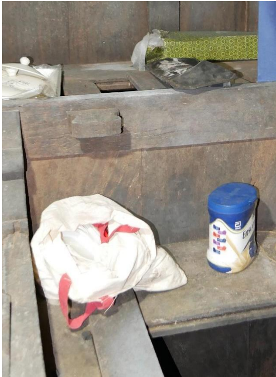
Figure 13. The various-sized openings on the surfaces in this wooden storage room, or ara , at one of the Vayattattil houses are where seeds or other precious goods were stored in the past. Image: JANAL Archives, 2024
