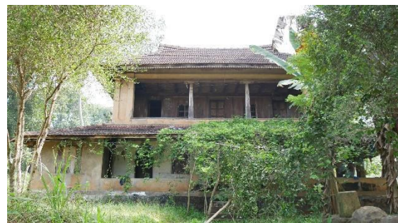
Figure 16. This two-storey house built for another ancestor of the Vyattattil family has only migratory workers from other states of India
