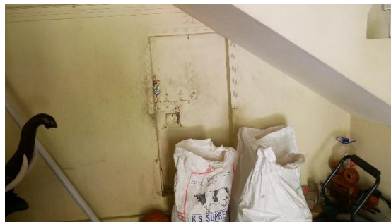
Figure 3. The door leading to an ara , the store room, where produce, seeds, and preserves were stored in the past. This ara , part of the original Vayattattil homestead, was built in the plot given by the Kaimals. It was retained when the house was demolished and rebuilt in the mid-20 th century. Image: JANAL Archives, 2024.
