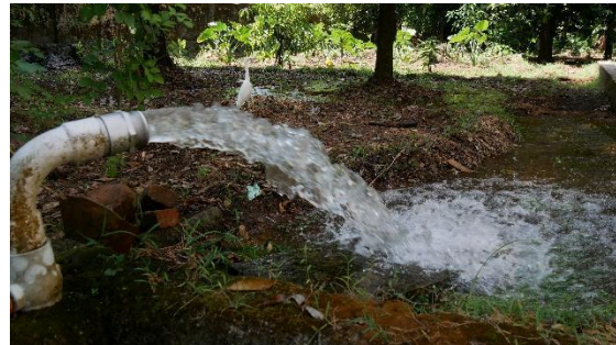
Figure 23. Water being pumped into the channels leading to the crops at Parakkadavu. Image: JANAL Archives, 2024.
